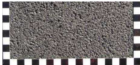
Thin layered asphalt
